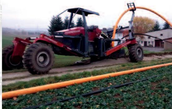
*Plowing in of a gas pipeline HDPE OD 180 and 2 x cable protection pipe OD 50.*
