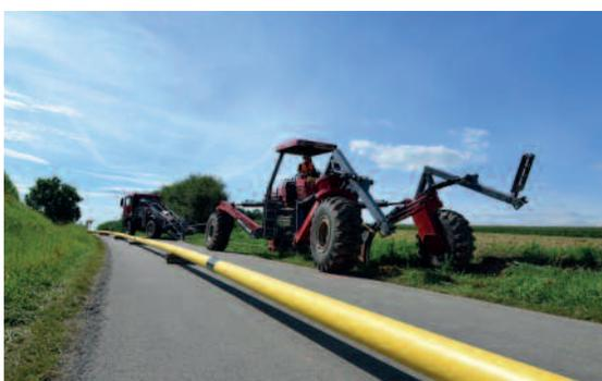
Surface after installing a drinking water pipeline 250 x 14.8 with the Rocket Plow.
