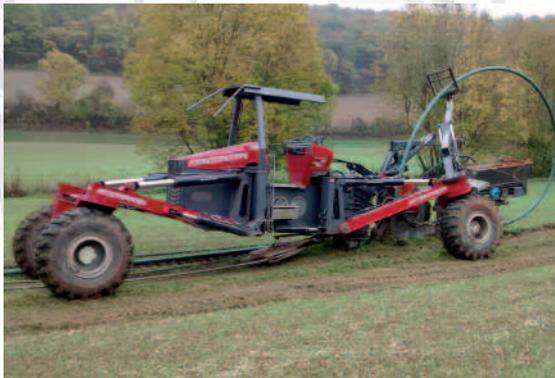
*Plowing in of a sewer pressure pipe HDPE OD 90.*
