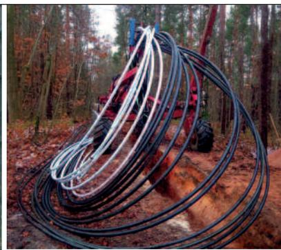
*Plowing in of 18 x cable protection pipe HDPE OD 50.*
