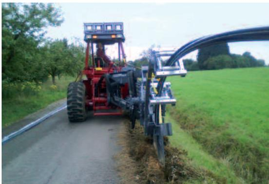
*Plowing in of a cable protection pipe HDPE OD 50.*
